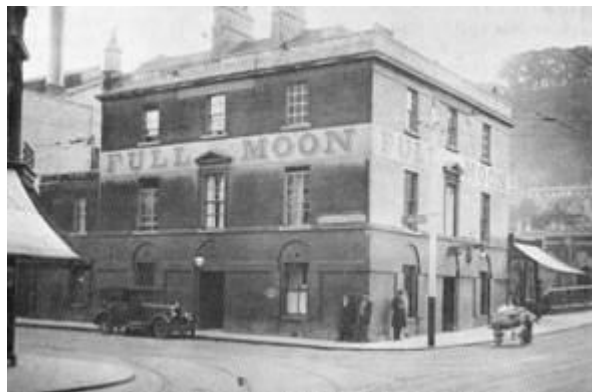
Fig.5 The Full Moon Hotel site of the new Showrooms and Offices (Courtesy Bath Reference Library)
